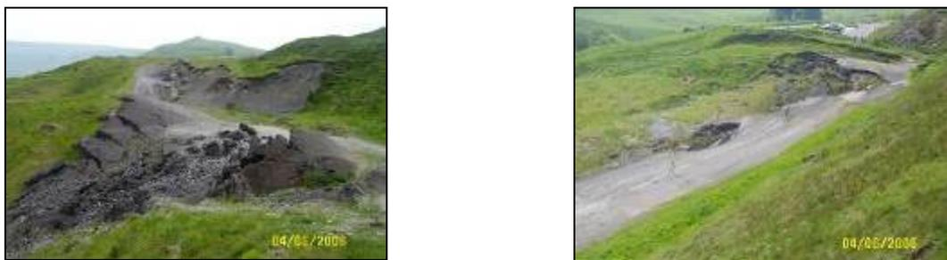
**Figure 6.** Severe damage to the A625 Manchester-Sheffield road which crosses the Mam Tor landslide. The road was finally closed to traffic in 1979 following repeated ground movements. Note the partly rotational slipped blocks with inward dips of up to 45°.
