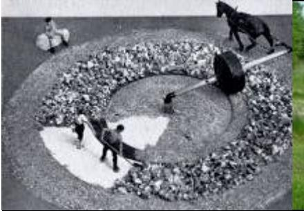
**Figure 2.** (Left) The Odin Mine crushing circle and wheel. Note that the crushing circle is now tilted and slightly buckled due to 'recent' movement on the landslide. (Right) Model of a crushing circle (model by H. E. Chatburn, H. M Parker, in Ford & Rieuwerts 1975).
