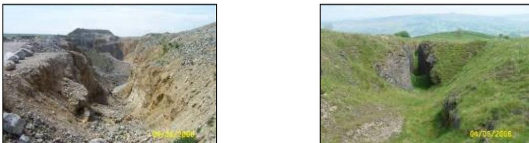
**Figure 14.** (Left) Open pit workings at Dirtlow Rake. (Right) Narrow 'gorge' caused by the historical, complete extraction of minerals in Dirtlow Rake.
