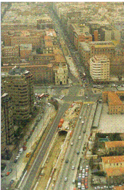
Figure 1. Aerial view of O'Donnell's tunnel
