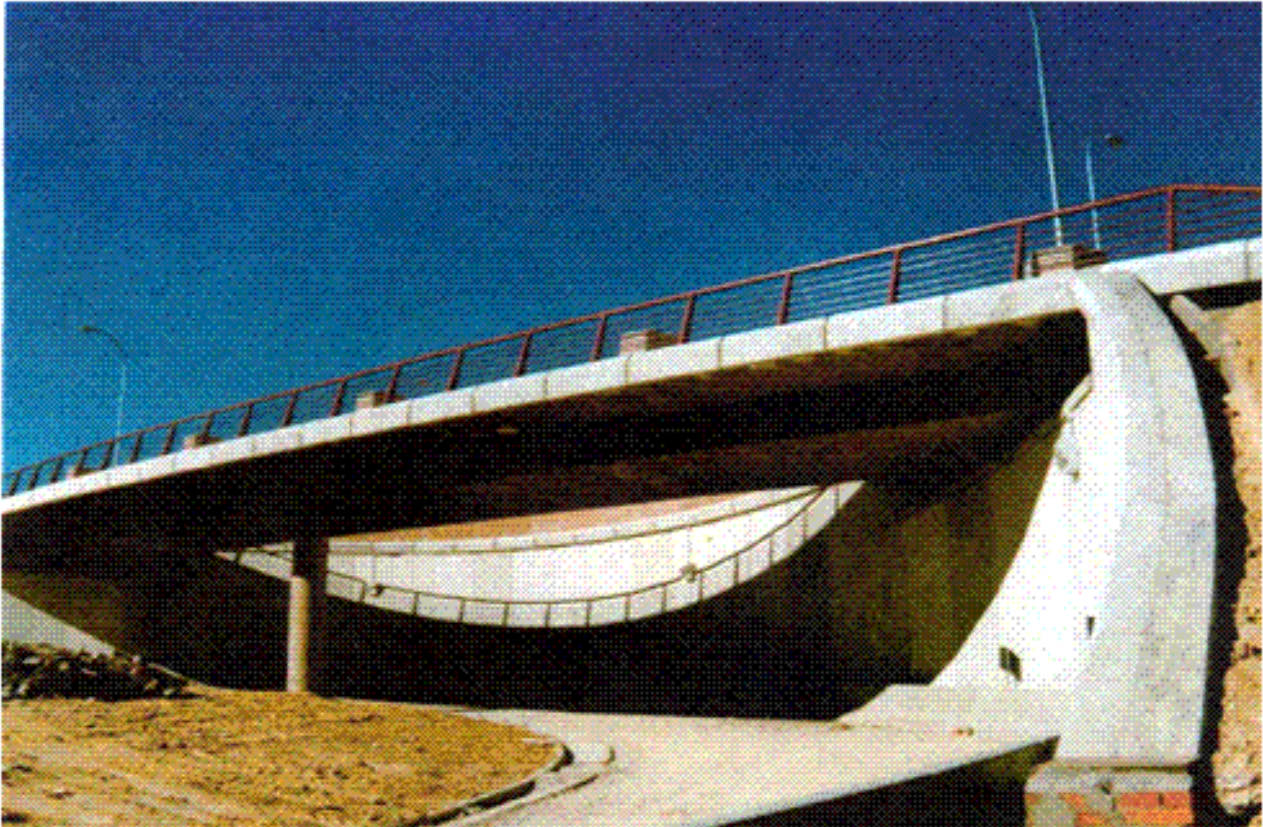
Figure 7. Bridge over the link to Alcalde Sainz de Baranda
