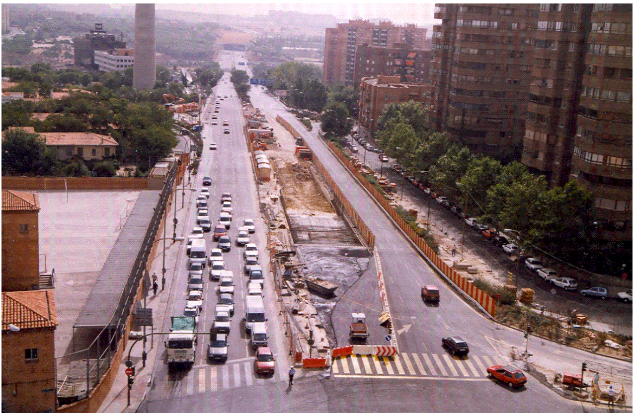
Figure 9. West entrance of the tunnel.
