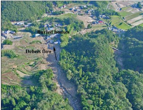
Figure 9. Buried village in Moriyeiki (see Figure 7 for location)
