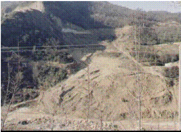
Figure 5. A view of landslide in downstream of Tajan dam
