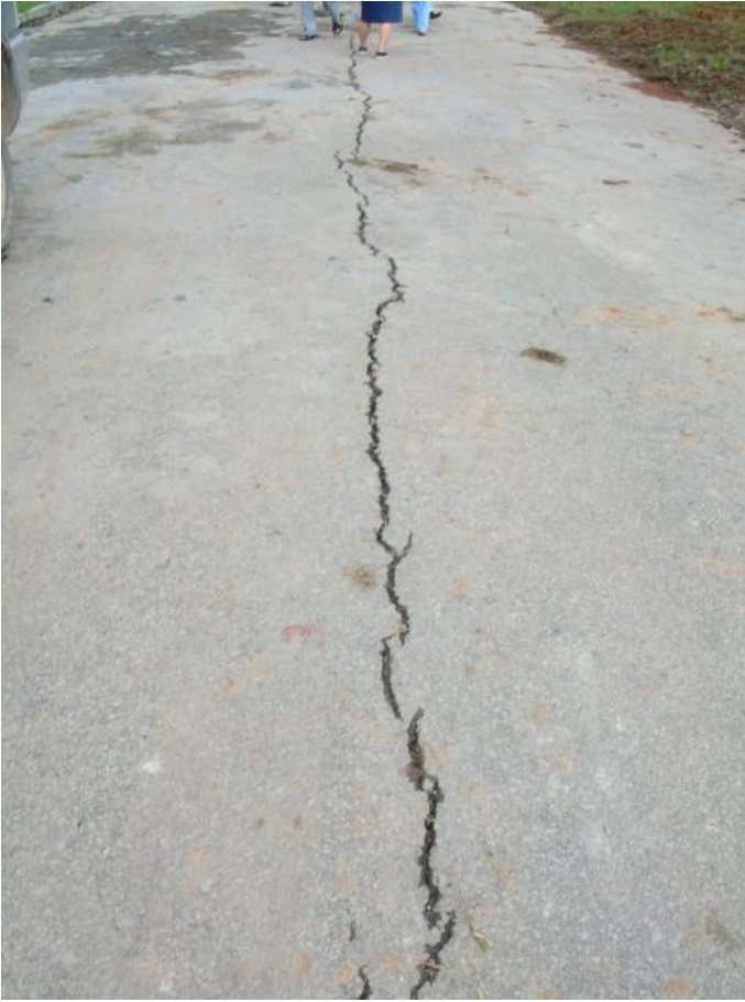
Figure 5. Crack at the crest of the fill slope showing horizontal displacement up to 100 mm
