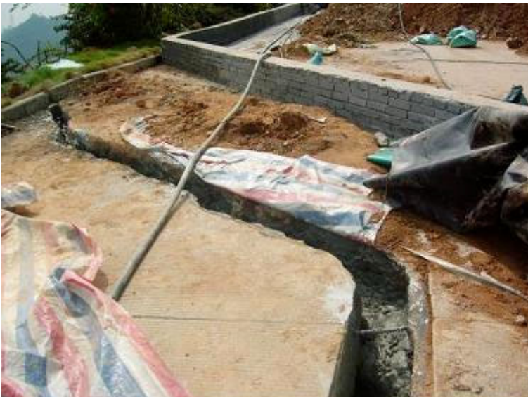
Figure 6. Crack on the berm of the fill slope showing horizontal displacement up to 500 mm
