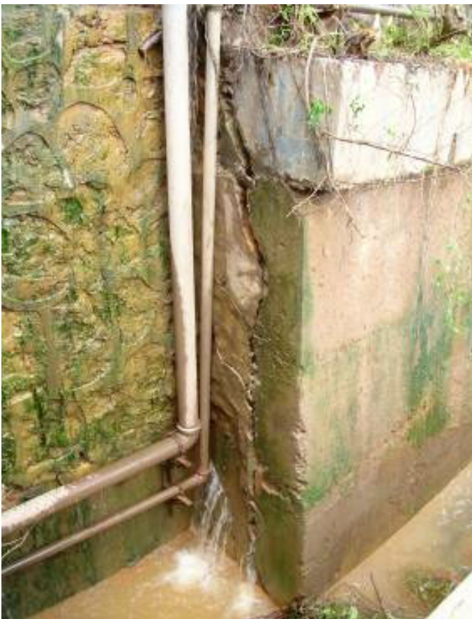
Figure 4. Vertical crack along the surface of the masonry retaining wall
