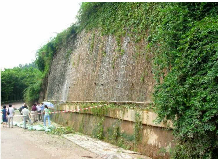
Figure 8. Groundwater flowing out of the weepholes of the masonry retaining wall
