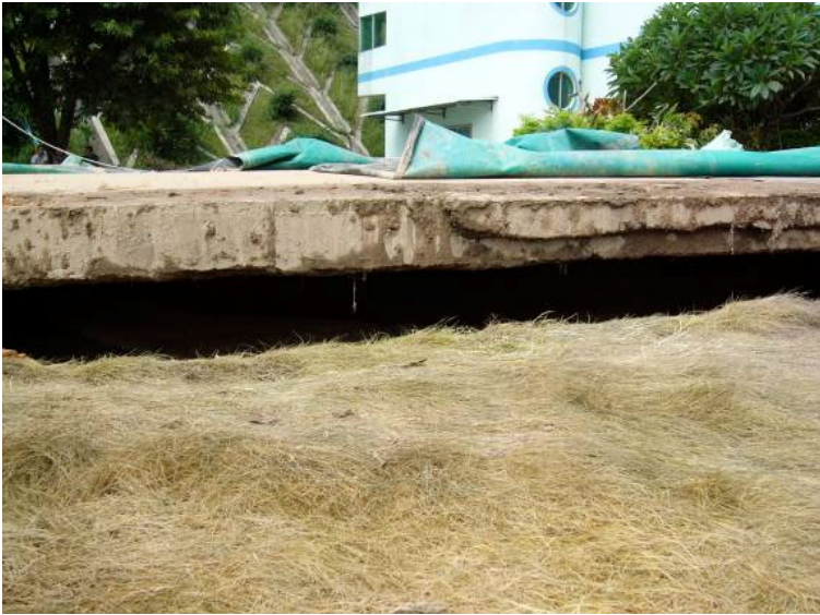
Figure 7. Soil under the pavement on the berm of the fill slope settled up to 500 mm
