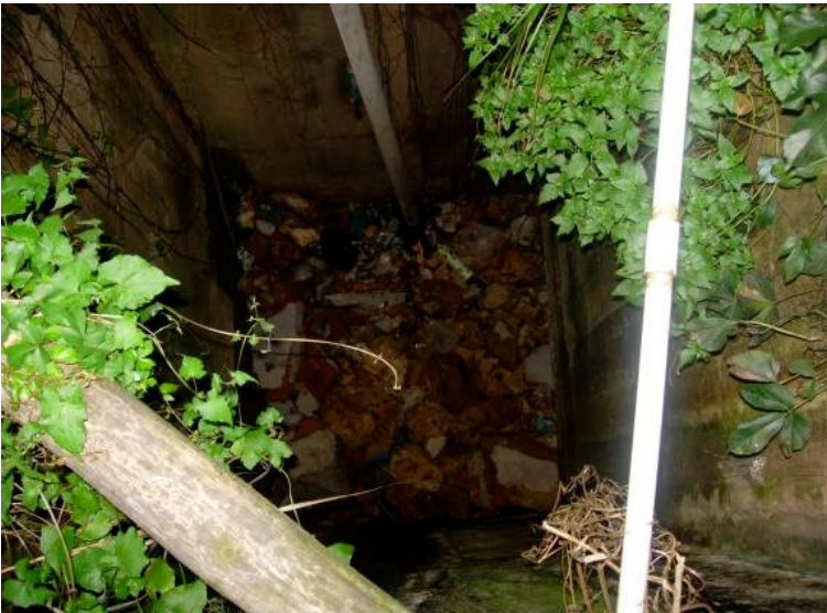
Figure 10. Drainage channel at the left crest of the fill slope was seriously damaged and blocked
