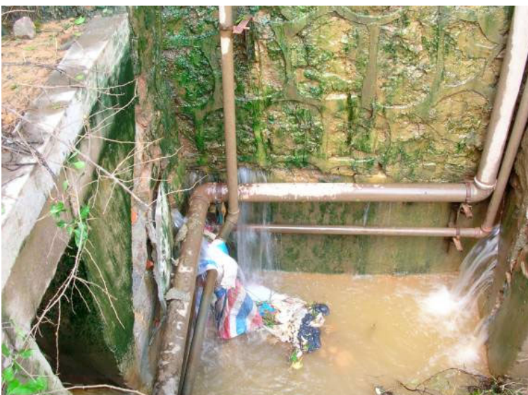
Figure 9. Groundwater flowing out of the cracks of the masonry retaining wall
