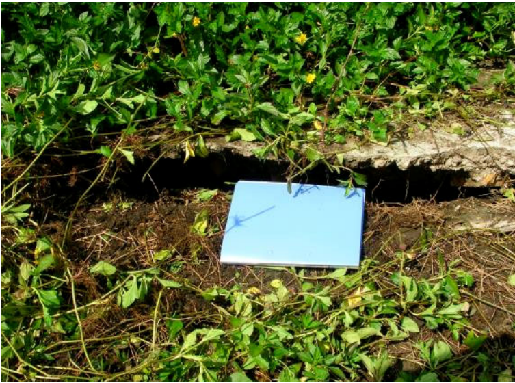
Figure 3. Crack on the top of the masonry retaining wall
