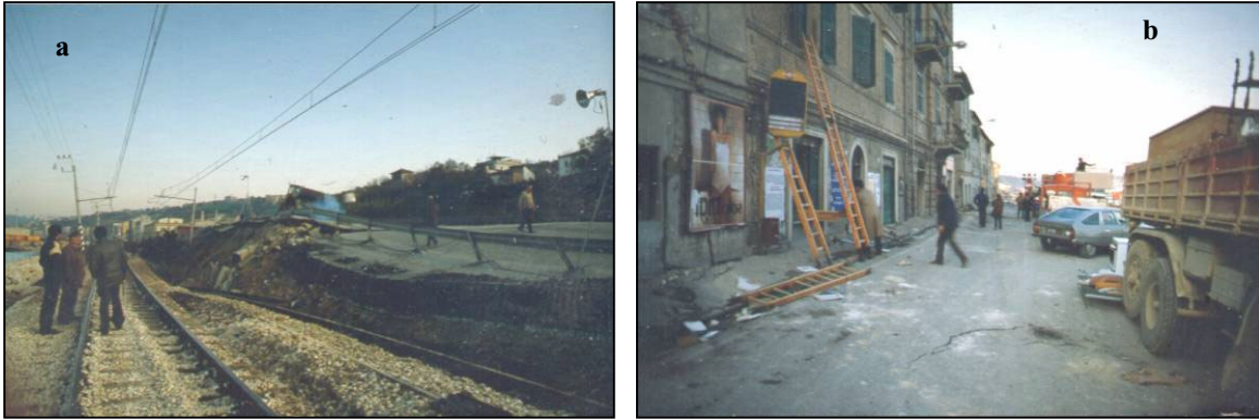
Figure 1. Railway (a) and Flaminia Road (b) interrupted by the landslide.
