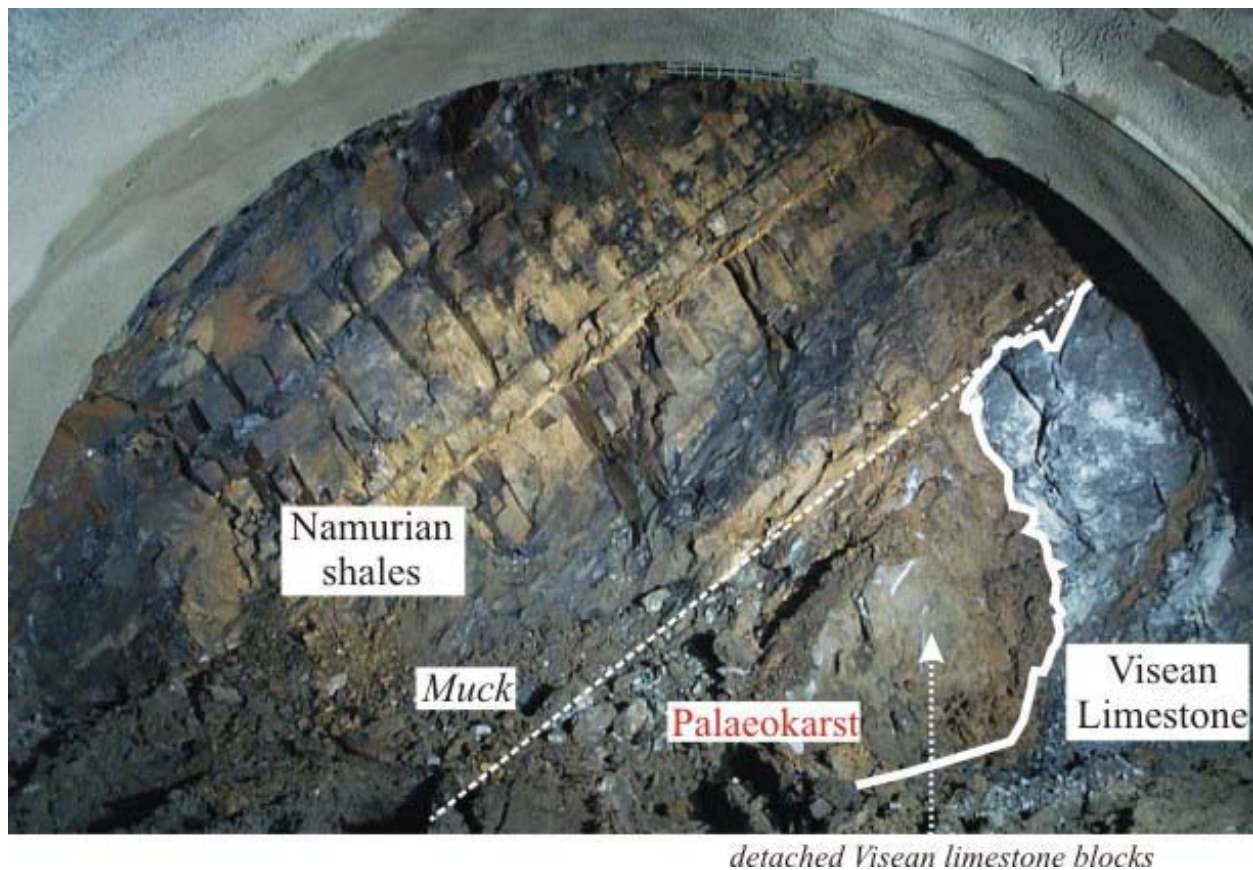
Figure 5. Tunnel front during the construction of the Soumagne tunnel (radius 5.5m) showing the palaeokarst on the Namurian-Visean interface (Photo: Courtesy of S.M. Soumagne Tunnel).
