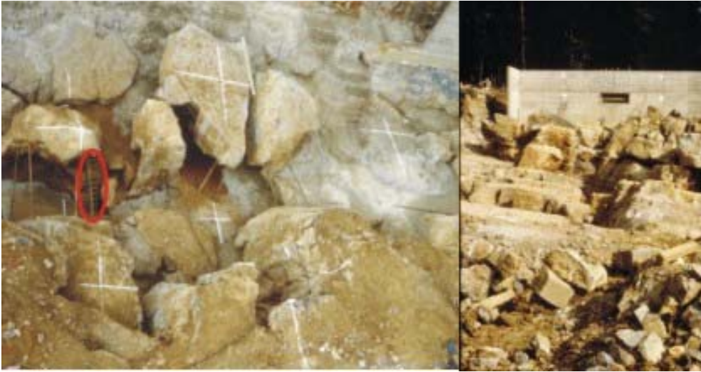
Figure 9. Mont Godinne construction site: The dimensions of the karst can be appreciated by the scale of the full size ladder encircled in red used by the working team to descend into the karst. Each white cross marks the points identified by the site investigation using the simple penetration test.
