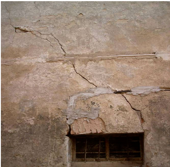
Figure 2. Fissure in the eastern front of Casa Wagner
