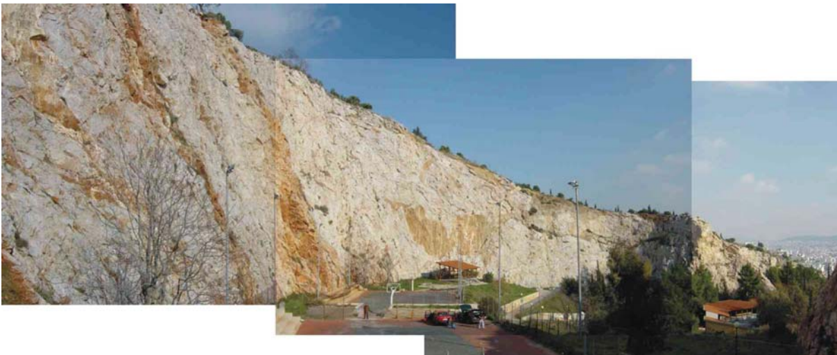
Figure 11. Panoramic picture of the slopes surrounding the sports fields. All the sports' infrastructures are located at the base of the slopes without keeping any safety distance.
