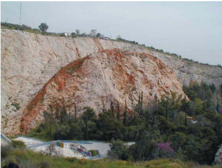
Figure 4. Extremely wide karstic fissure (up to 15 m) filled with clay materials. The material has enclosed blocks of the Turkovounia limestone. During the excavation the surrounding limestone was untouched in order to avoid moving the enclosed materials.
