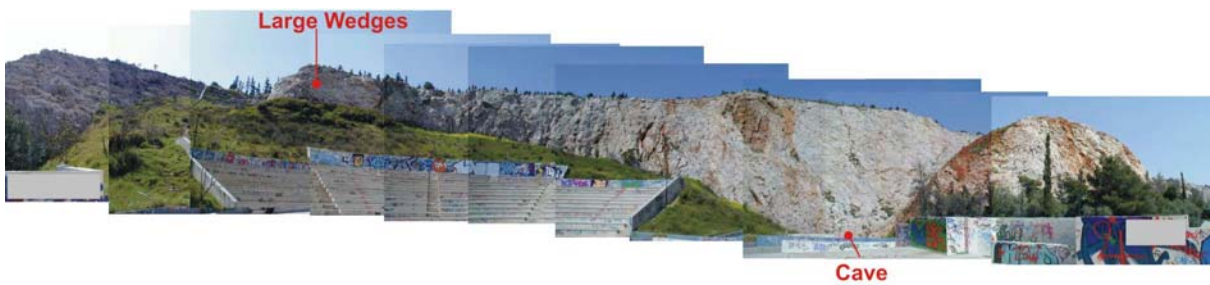
Figure 7. Panoramic picture of the slopes surrounding theatre. The notes point out the section of the slope with the large wedges and the location of the cave presented in Figure 5.
