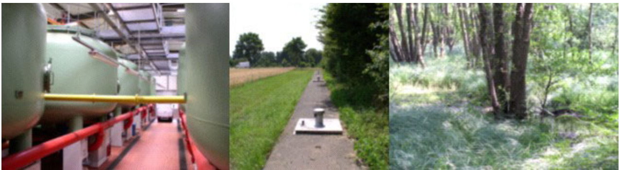
Figure 9. Water pumped in the vicinity of the Garzweiler mine is pumped to the eco-water treatment plants on the left. After treatment the water is pumped to infiltration trenches and infiltration wells. In the middle an infiltration trench is shown. These infiltration trenches guarantee a high water table for the wetlands shown on the right.
