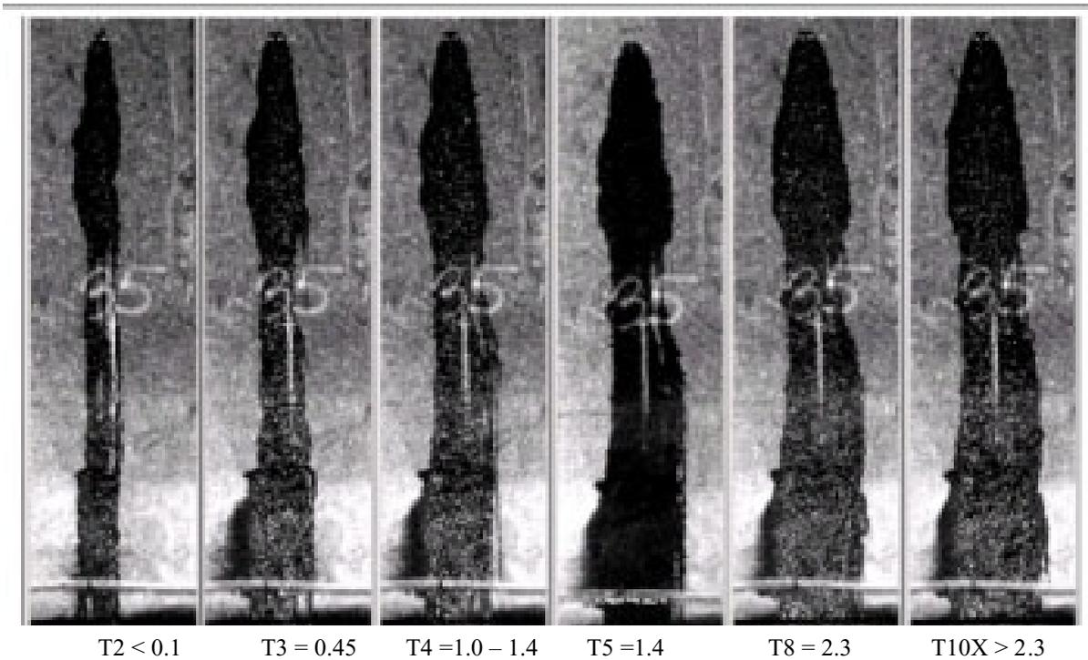
**Figure 6.** Different water leakages shown as a grey-scale image of the TBM tunnel wall
