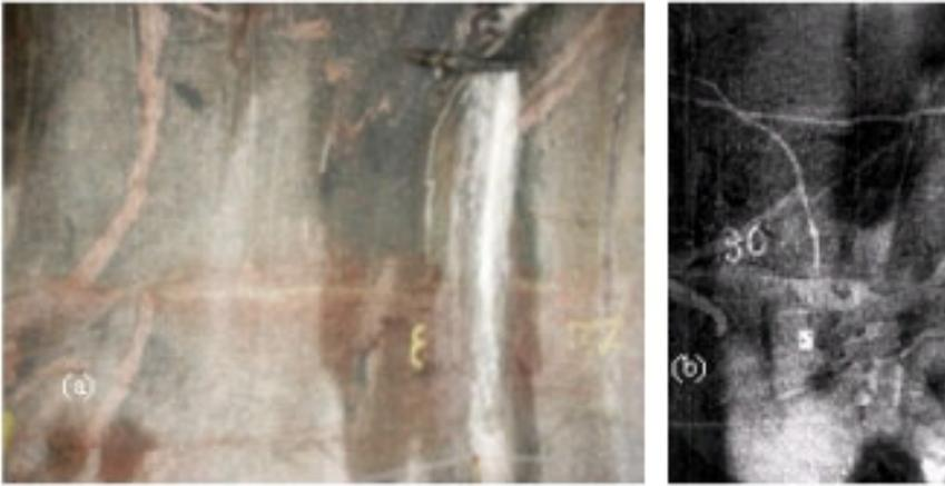
**Figure 5.** Water leakage showing in both photo (a) and laser image (b)
