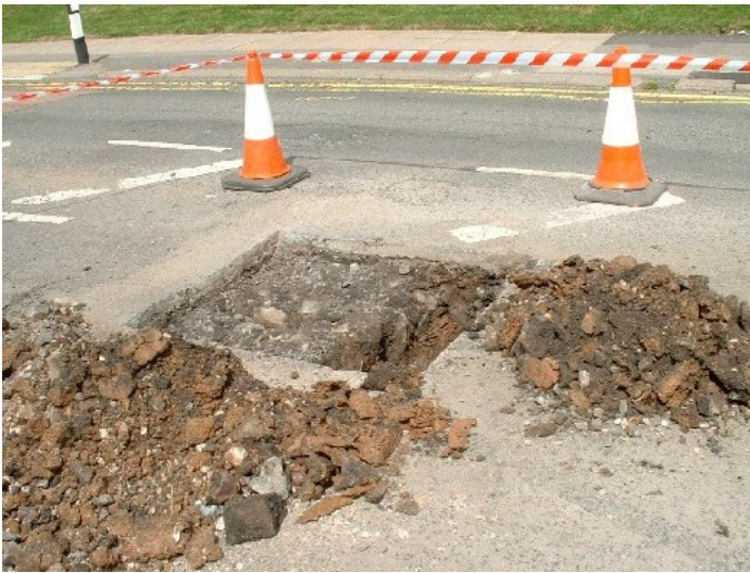
Figure 2. Trial pit showing bituminous road pavement, pitchings and silty clay subgrade
