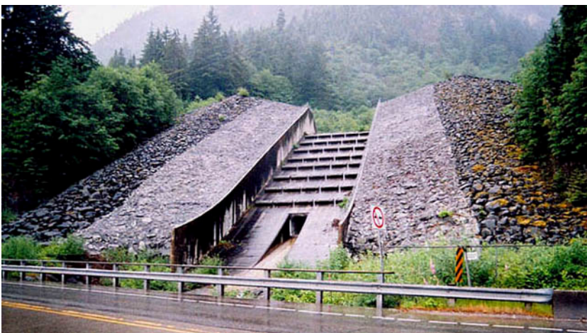
Figure 8. Concrete spillway on the downstream face of a debris basin barrier, Charles Creek, Sea-to-Sky Highway, BC, Canada. The drainage outlet may be seen in the centre of the spillway.
