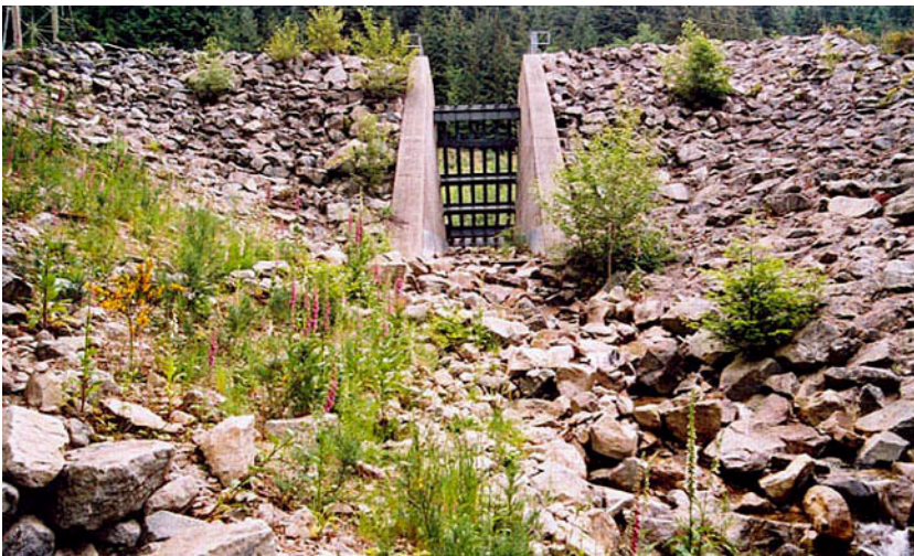
Figure 7. Debris basin showing the downstream barrier and drainage outlet, Mackay Creek, N Vancouver, BC, Canada.
