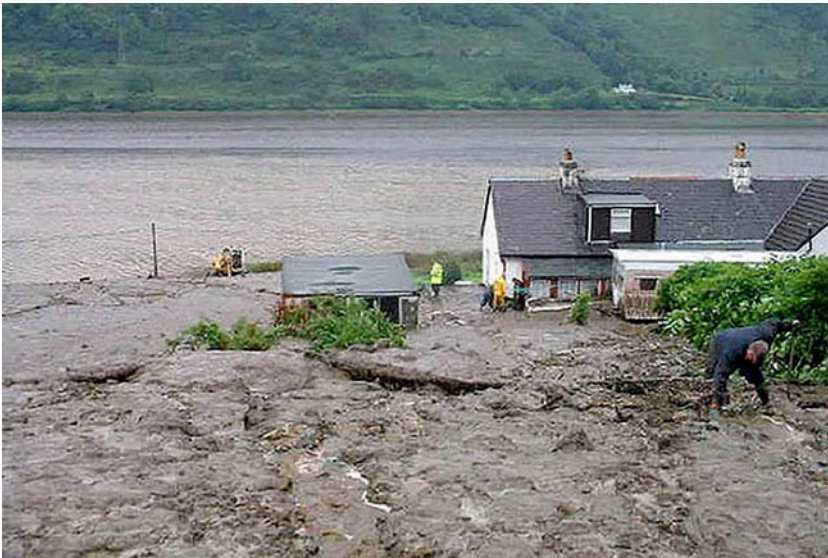
Figure 3. A83 debris flow to the west of Cairndow showing the effects on a roadside cottage and the trunk road immediately downslope from the cottage.
