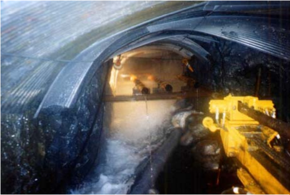
Figure 1. A situation of drainage countermeasure in the tunnel
