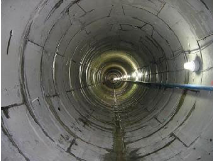
Figure 2. Assembled PCTL Segments in a Tunnel
