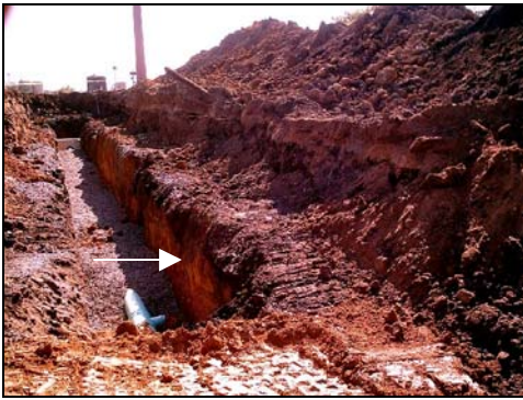
Figure 4: Sanitary sewer installation at The village of Rockets Landing. Fill contaminated with coal combustion byproducts visible above arrow. The pipe in the foreground is 0.3 meter diameter.
