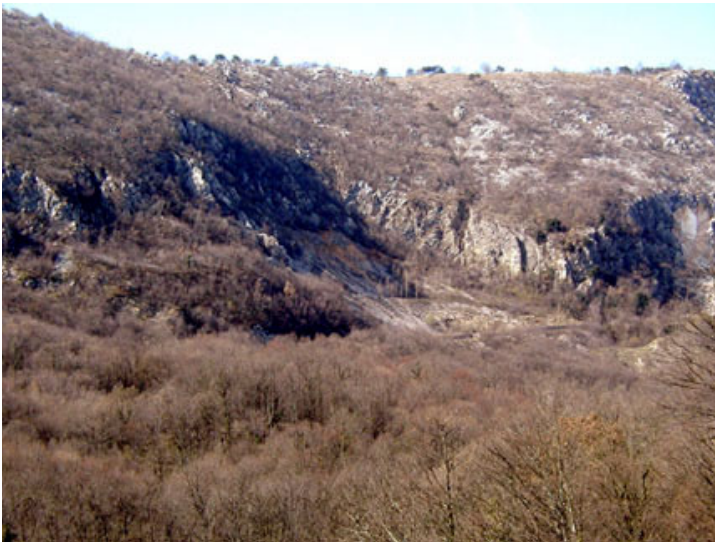
Figure 4. Debris avalanche and rock slide on SW slope of river valley, marked as A on Figure 2
