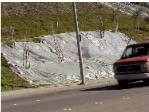
Figure 1. Translational landslide on landscaped slope
