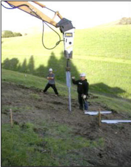
Figure 4. Installation of a plate pile with a modified hoe-ram attachment on an excavator
