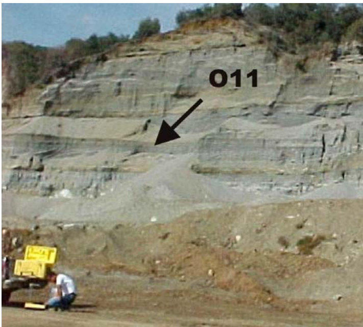
Figure 3. Unstable slope O11, between ch.20+500 and ch.20+800
