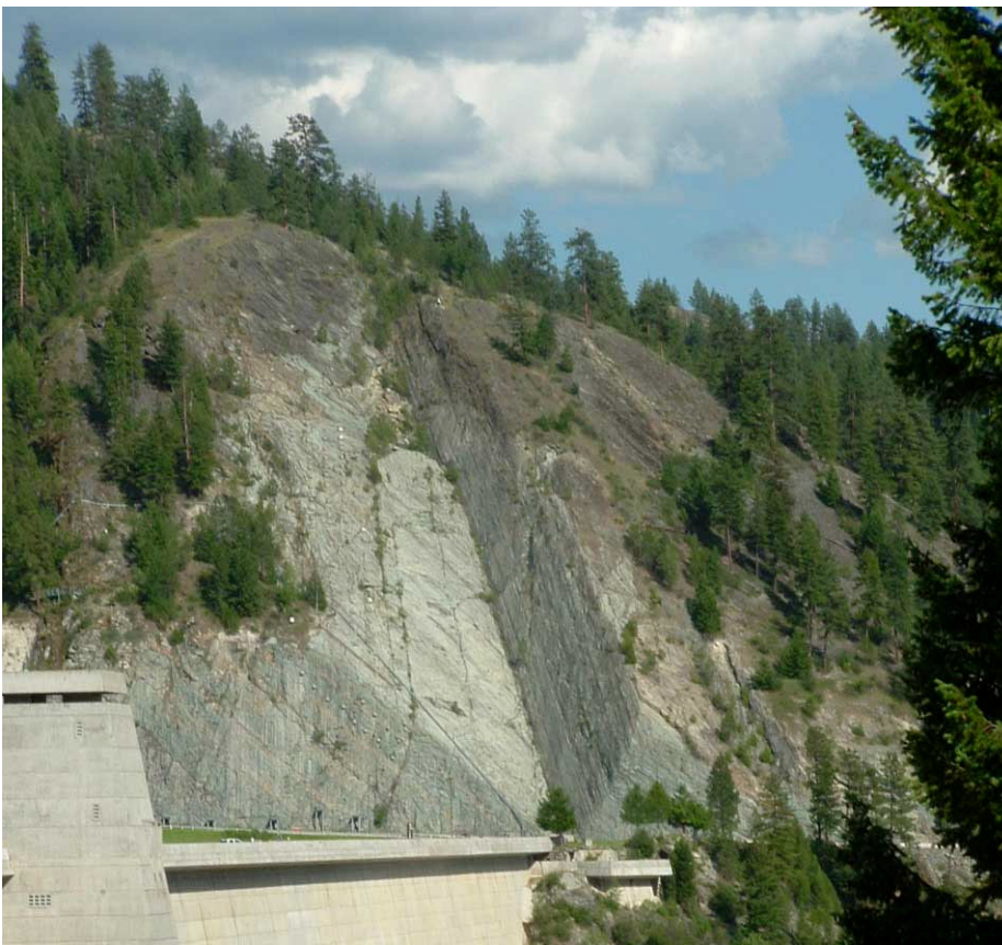
Figure 1. Today's appearance of the mitigated remains of the “Dirty Shame” rock slide of 1970, located at the immediate left abutment of Libby Dam, northwest Montana. This failure occurred during construction and was unanticipated in the course of collection and evaluation of site geologic observations and rock structural data and constitutes a major “lesson learned” in the annals of American engineering geology. The remaining failure trough speaks eloquently for the geologic character of the bounds and properties of the pre-failure rock mass. There were no fatalities. (Image by the author, 2005)
