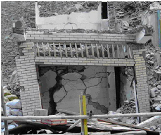
Figure 3. The destroyed houses in the leading edge of the landslide
