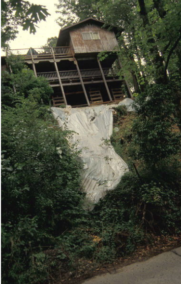
Figure 4. Earthflow in the West Hills began where a gutter deposited water (Burns et al. , 1998, Slide #119)
