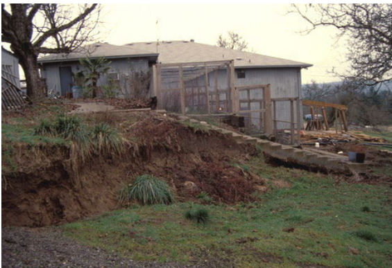
Figure 7. Ancient landslide in the Troutdale Fm drops one metre (Burns et al. , 1998, Slide #272)
