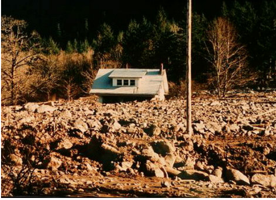
Figure 10. Debris flow buried the Royse homestead, Dodson, Columbia River Gorge (Burns et al. , 1998, slide #128)
