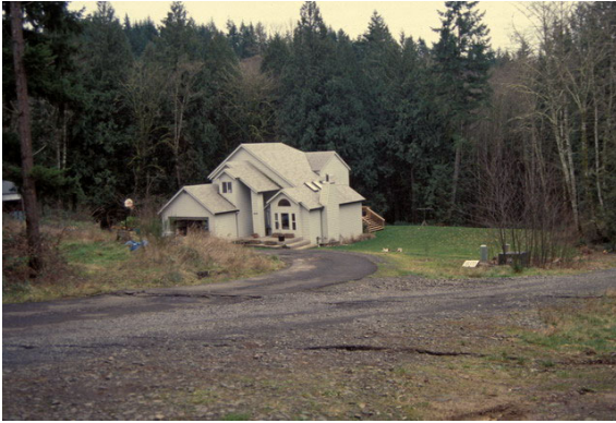
Figure 6. Toe of ancient landslide moves 0.3 metres laterally and causes distress for house (Burns et al. , 1998, slide #263)
