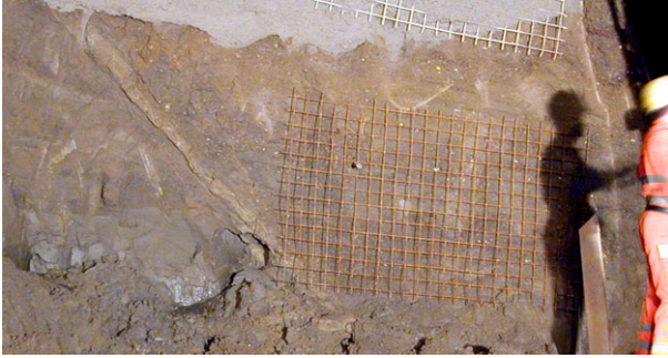
Figure 3. Fault between silty grey sand (left) and brown sand (right). The right hand side is displaced downward for more than 12 m. The fault is filled with silt. So the fault works as a barrier to groundwater. Seepage occurs in the silty grey sand where the groundwater is dammed up.
