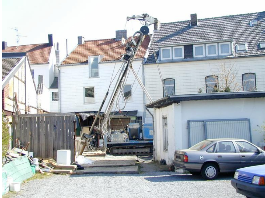
Figure 8. Inclined boring on a shaft with adjacent residential housing
