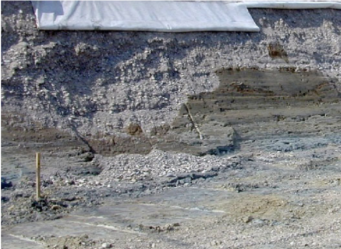
Figure 4. Holocene fluvial gravel channel incised into Neogene finegrained soils. Slope of excavation pit north of Munich (slope is 4 m high)
