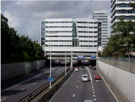
Figure 7. The Equinox building above the Utrechtse Baan in Den Haag
