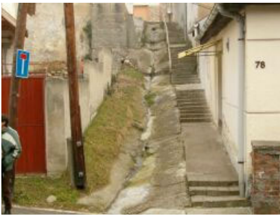
Figure 5. Precipitation drainage ditch (Pécs)
