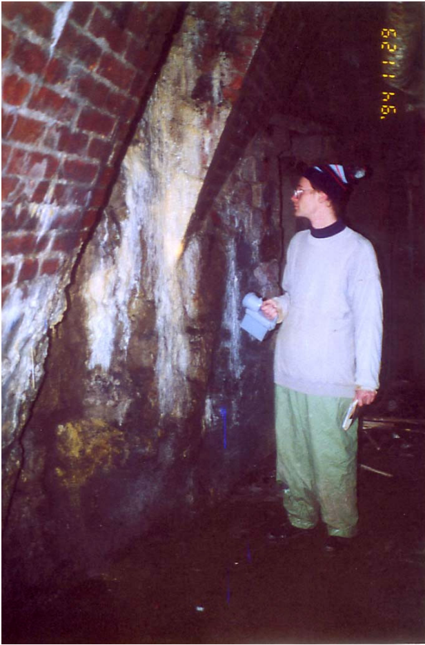
Figure 7. The cave system of the Castle Hill of Buda, water inflow deriving from the defect of public utilities
