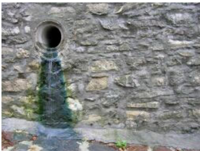
Figure 2. Periodic water overflow in a retaining wall (Veszprém)
