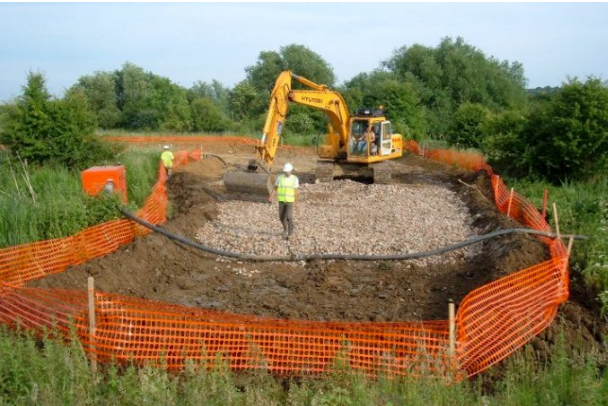
Figure 6. Construction of piling platform for groundwater barrier within sensitive wildlife areas
