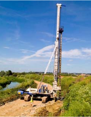
Figure 5. Photograph of in-situ soil mix barrier installation
