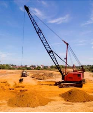
Figure 8. Photograph of dynamic compaction rig
