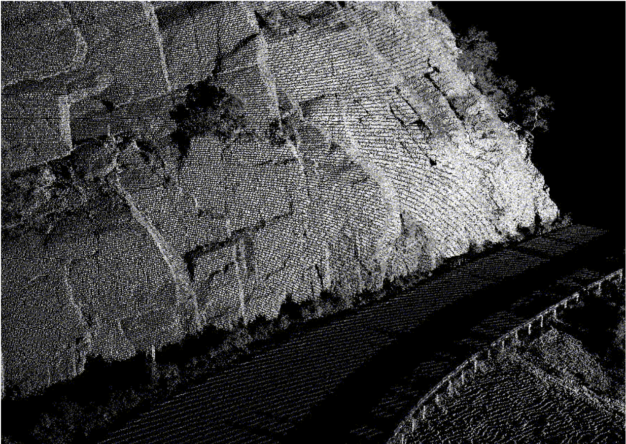
Figure 1. A typical point cloud representation of a highway rock cut. Visible rock cut is about 10 meters high.
