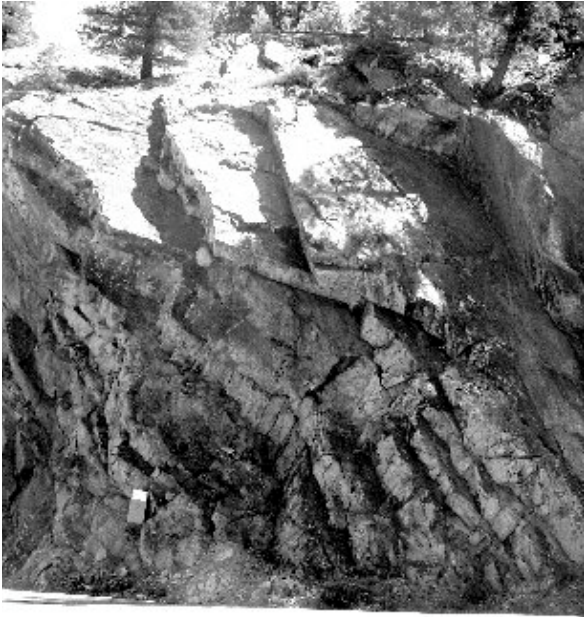
Figure 8. Colorado rock slope Photo 1. Height of view about 8 meters. At this exposure, several joints and foliations form prominent exposed surfaces.
