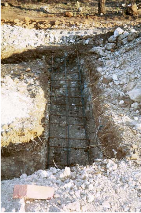
Figure 2. Reinforcement in shallow foundation.
