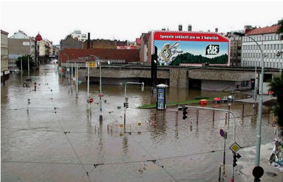
Figure 7. Flooded Florenc Metro Station
