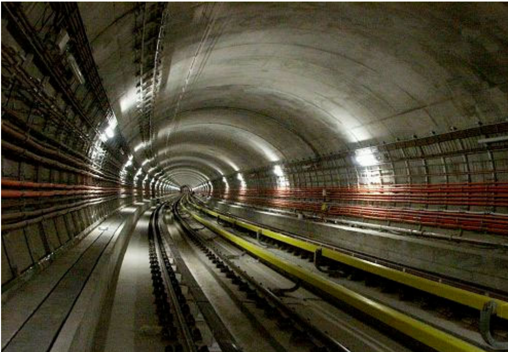
Figure 2. Double-track Metro tunnel on line IV.C
