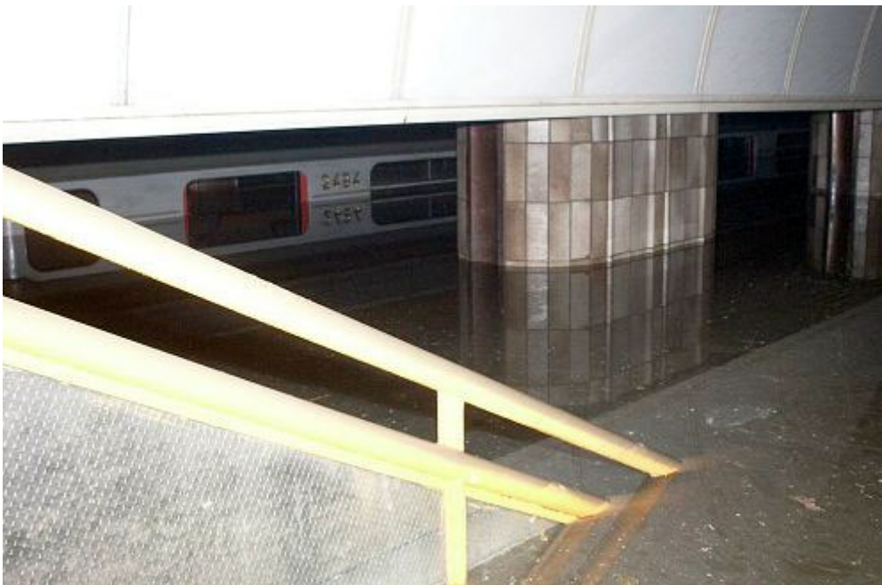
Figure 8. Submerged metro train in Florenc Station
