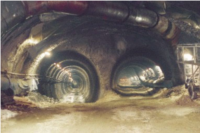
Figure 12. Construction stage of İstanbul Metro
