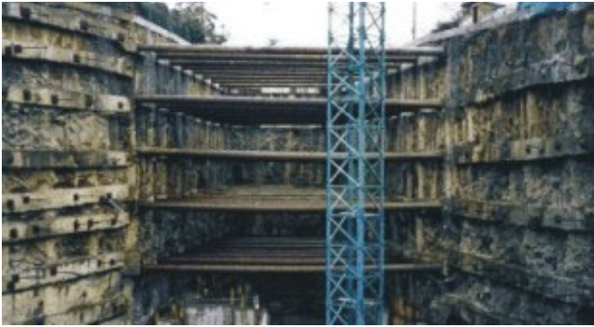
Figure 9. Foundation excavation in graywackes
