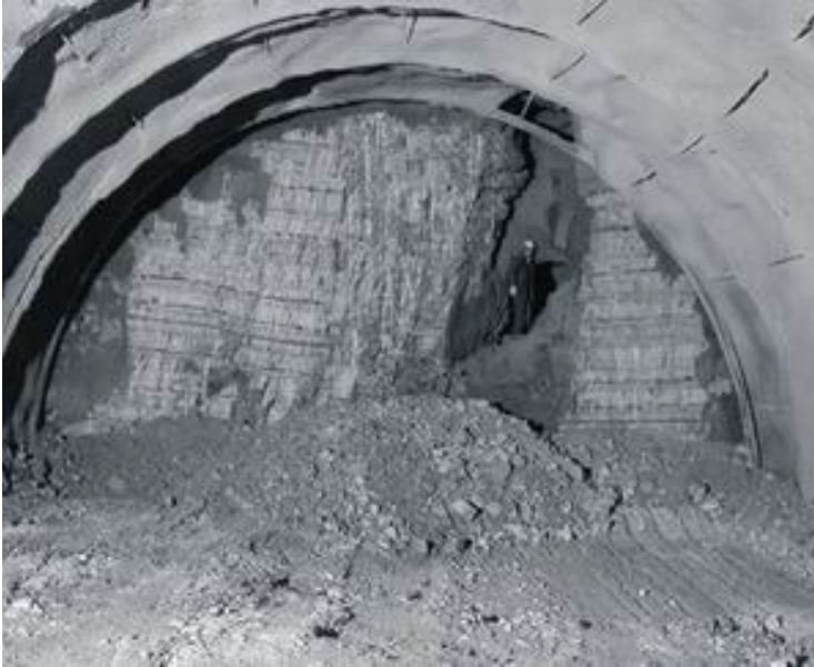
Figure 4. Typical appearance of a small karstic void partially filled with clay and silt; Dodoni tunnel, northwestern Greece, 2000.
