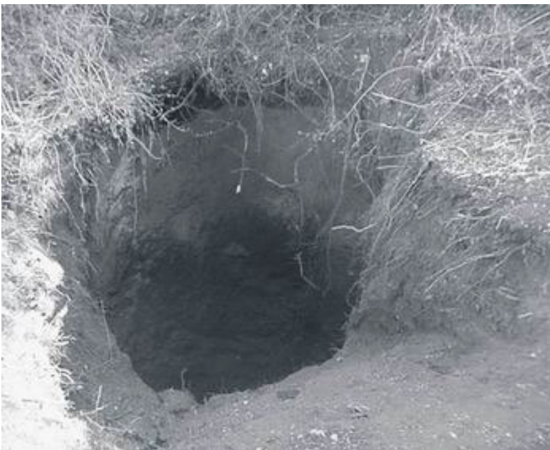
Figure 5. Collapse of the filling of a karstic chimney crossed by Dodoni Tunnel. The collapse outcropped on the surface at about 100 m. over the tunnel
