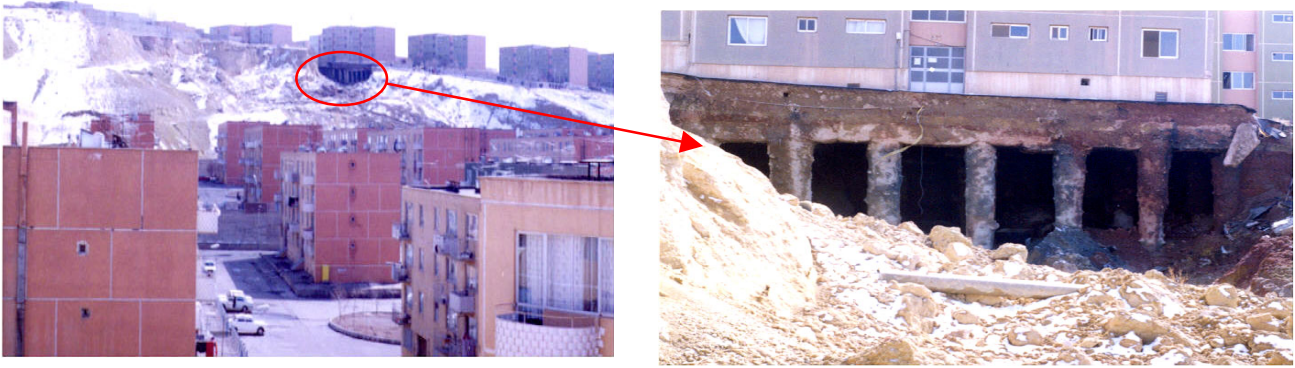
Figure 13. Mud flow type slide occurred in Tabriz Marl
