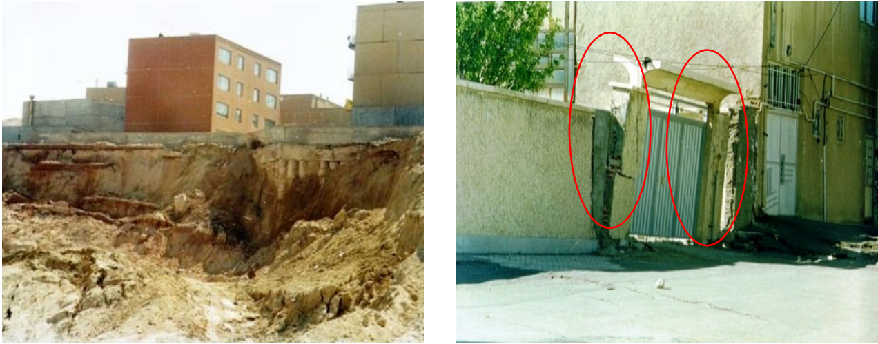
Figure 2. Construction on a fill area and large settlements and slides
