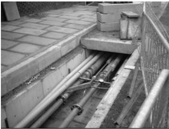
Figure 10. CHP pipes at the University of Birmingham
