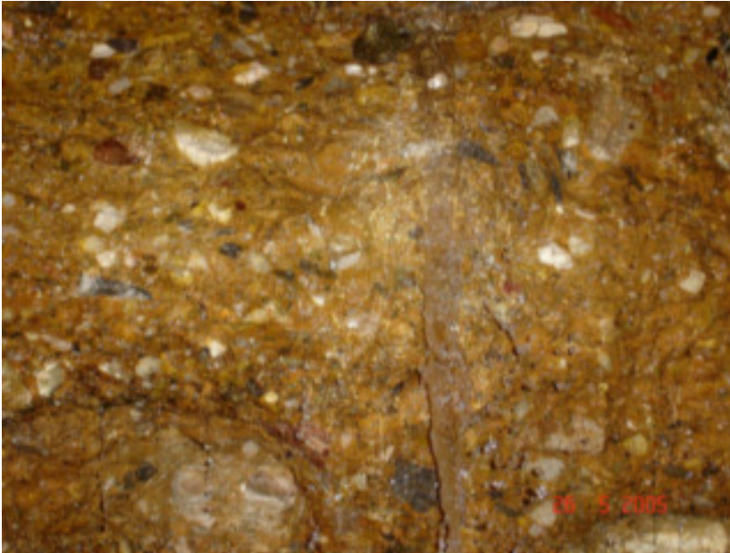
Figure 10. Water flow through the conglomerates of the old river bed at the tunnel face.
