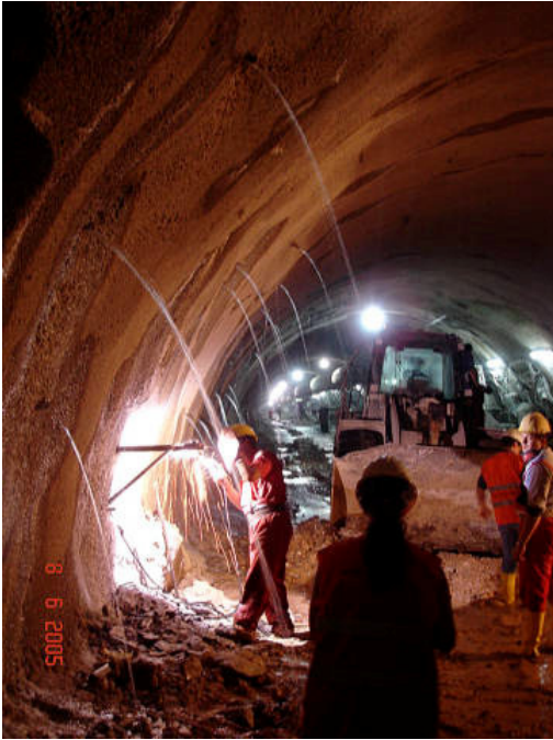
Figure 12. Water inflow from the tunnel side through drainage holes at the area of the old river bed.
