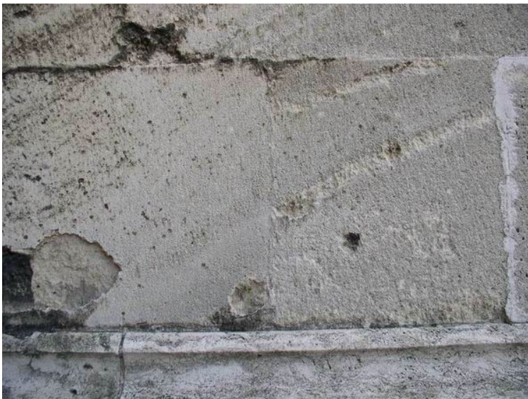
Figure 5. White scaling weathering crust on oolitic limestone
