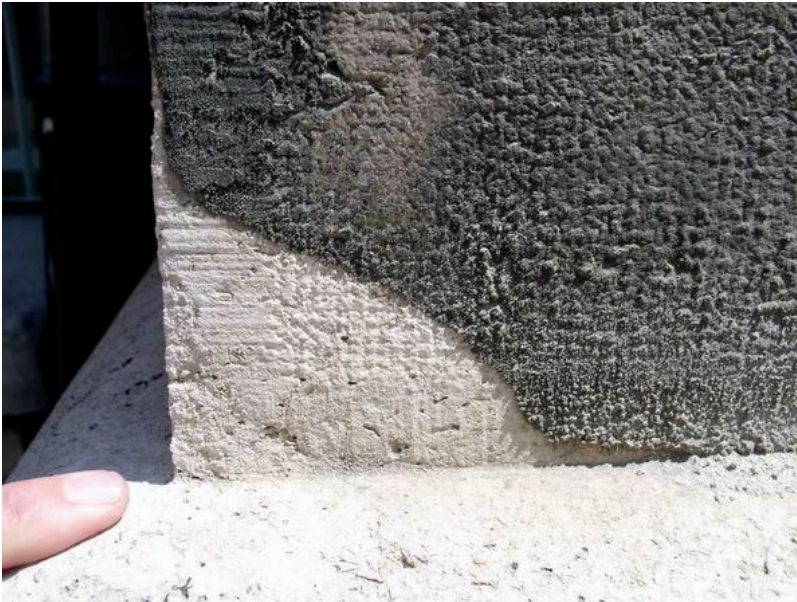
Figure 2. Black framboidal weathering crust on travertine
