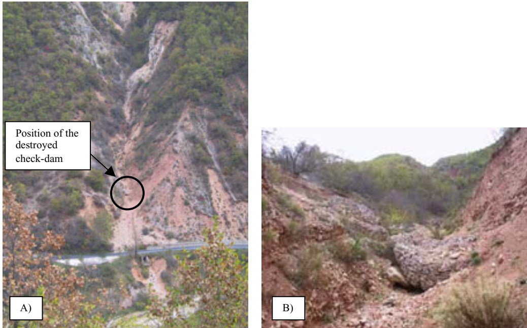
Figure 5. A) Final part of the San Giorgio creek, cut by the state road; and B) image of the check-dam destroyed by the debris flow.
