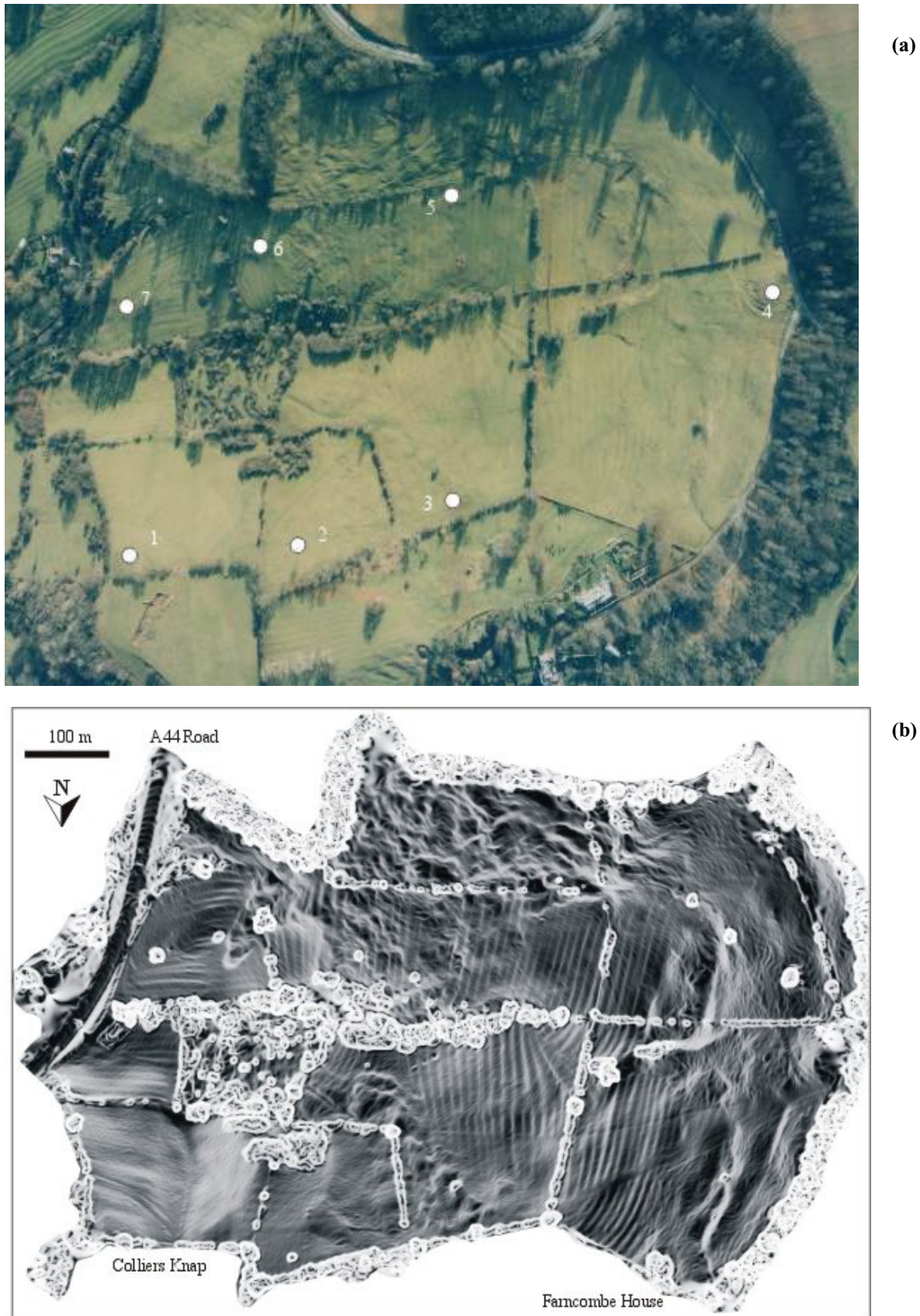
Figure 2. (a) Colour aerial photograph of the Broadway valley site indicating the location of each of the laser scan sites and the nature and extent of the slope instability. (b) Slope angle map derived from the digital elevation model of the Broadway valley generated using terrestrial laser scanning (resampled to 1 m grid spacing). In this image the steepest slopes appear white and are associated with landslide scarps and boundaries, frontal lobes and the top of the woodland canopy and hedge boundaries.
