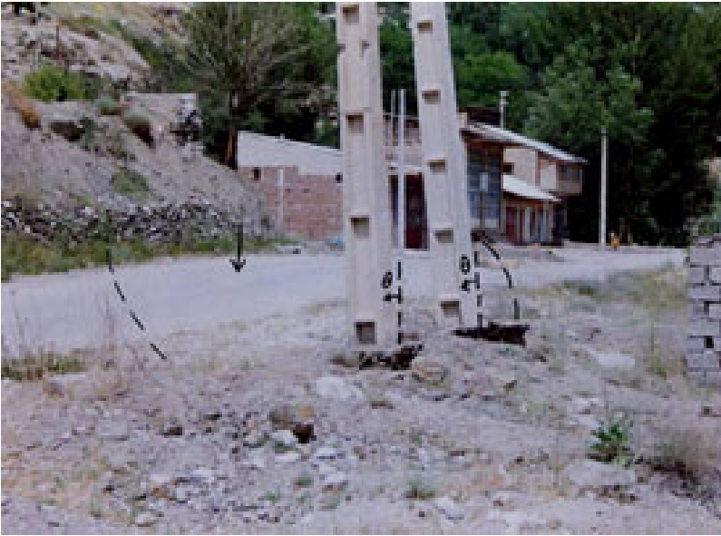
Figure 4. Inclination in power transmitting line at the toe of the slide
