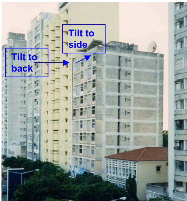
Figure 4. Site 1, Avenida Julius Nyerere
