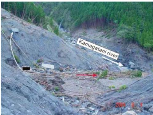
**Figure 13.** A displaced concrete block from the soil-conservation (Check) dam on the slope opposite the landslide source (Black area outlined by the broken white line: former location of the block; Red arrow: the flow direction of the valley water; White curved arrow: the move direction of the block)
