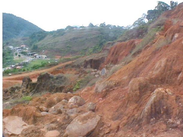
Figure 6. Example of an environmentally degraded site. Semi-active mineral exploitation contributing to hazardous conditions due to potential instability.
