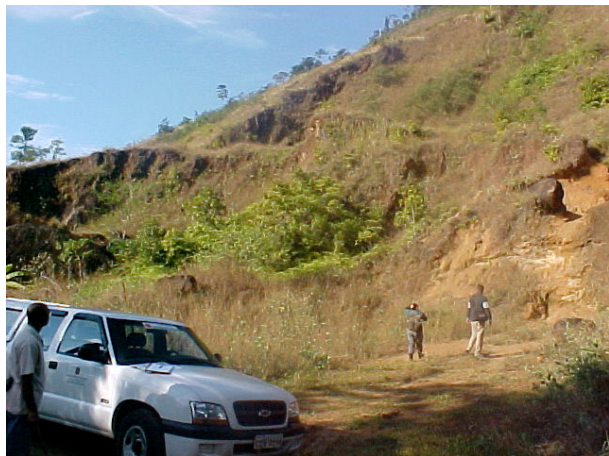
Figure 8. Example of an abandoned, partially recovered site. Note hazardous area due to ground instability, close proximity of road, and potential for occupation by low income populations.
