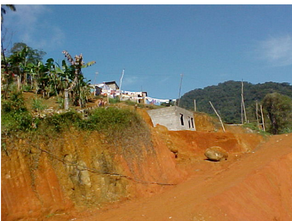
Figure 9. Example of unsightly and environmentally degraded site with potential for mineral exploitation of residual soil. Hazardous area due to declivity, ground instability (note detached blocks of rock), and informal occupation by low income populations
