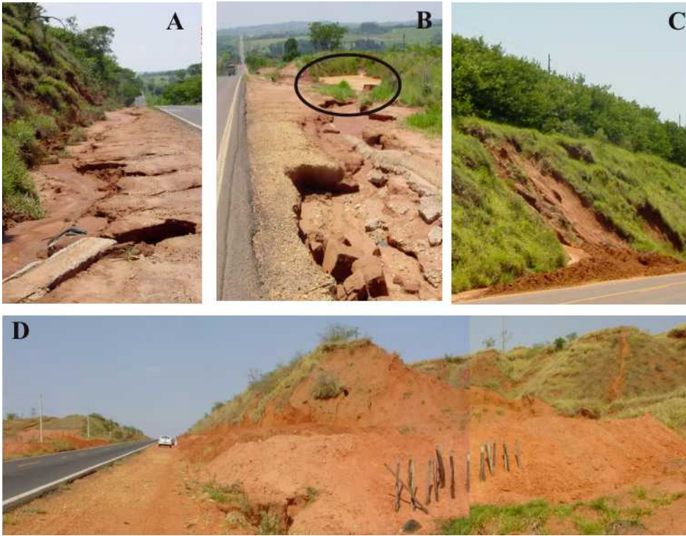
Figure 9 - Slope and road affected by erosion process (a- ravine, b- control measure, c- slipping and d- gully).
