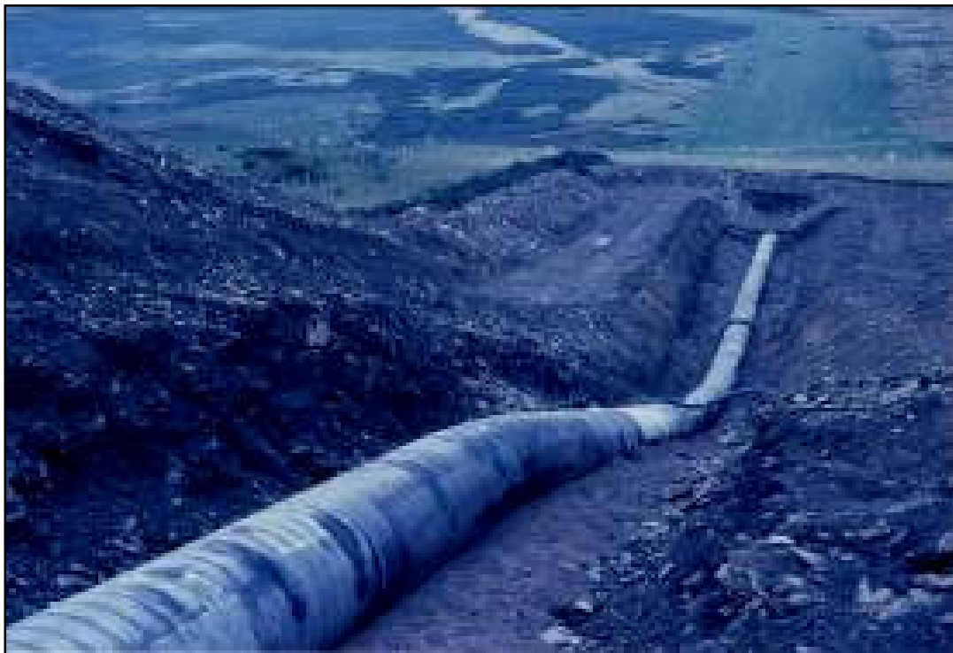
Figure 8. Influence of fault reactivation on gas mains. The Nelson to Dowlais gas main, exposed for strain accumulations and subsidence monitoring where it crossed the Rhos Fault, South Wales, UK.
