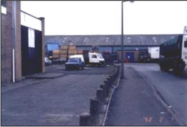
Figure 3. Lateral shear along the outcrop position of the Hollybush Fault, Staffordshire, UK. Note the 0.1 to 0.3 m of shear displacements to the kerbstones, paving slabs and the building's wall.
