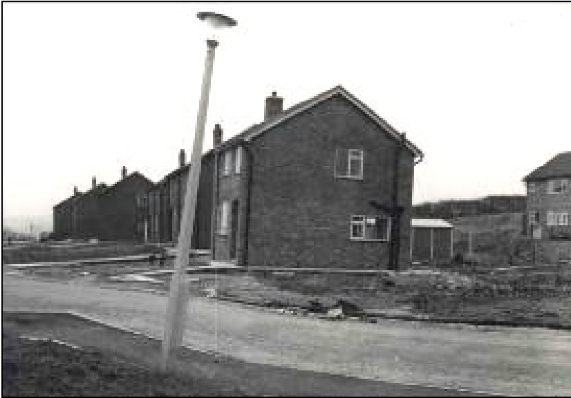
Figure 10. Reactivation of the Apedale Fault, in 1963, causing tilt to a lamp post, (note the vertical string hanging from the lamp post), Knutton, Staffordshire, UK
