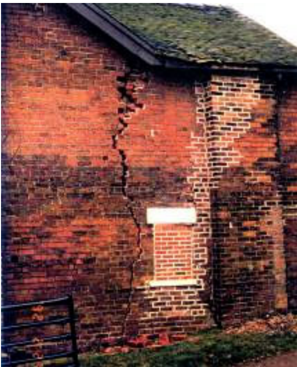
Figure 1. Damage to houses caused by the mining-induced reactivation of the Hopton Fault, Oulton, Staffordshire, UK.
