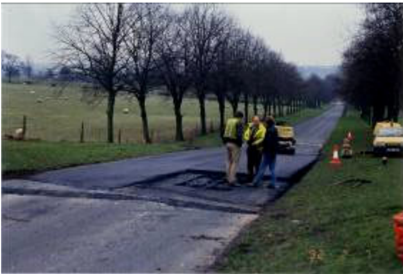
Figure 6. Repairs to Wedgwood Drive, Barlaston, Staffordshire, UK, caused by the reactivation of the Crowcrofts Fault. This generated a scarp at least 1.0 m high and 1.5 km long, during multiple phases of reactivation from the 1960s to 1990s.
