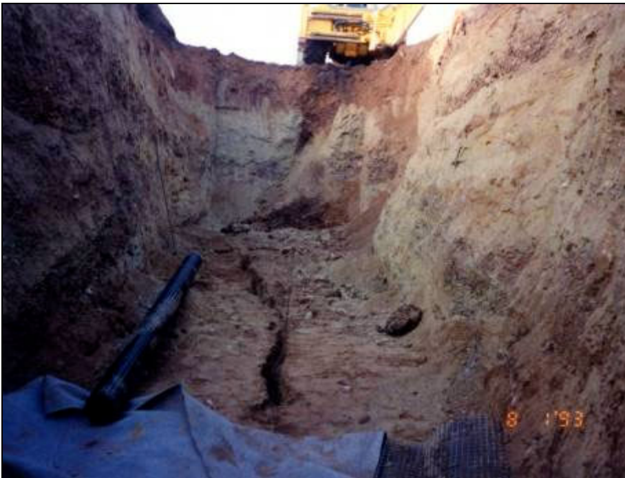
Figure 9. Fissuring associated with the reactivation of a fault, Downes Bank, Staffordshire. This caused disruption to underground communications cables. The fault is exposed in a trench and the ground stabilised using a geotextile mesh and granular fill.
