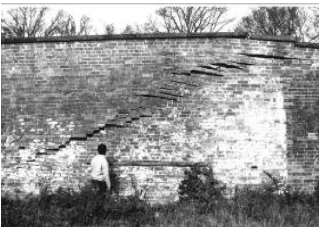
Figure 5. Compression to a 5.0 m high retaining wall, caused by fault reactivation and subsidence, Eastwood Hall, Nottinghamshire, UK.
