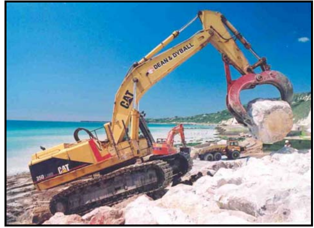
Figure 13. Rocks are placed at low water.
