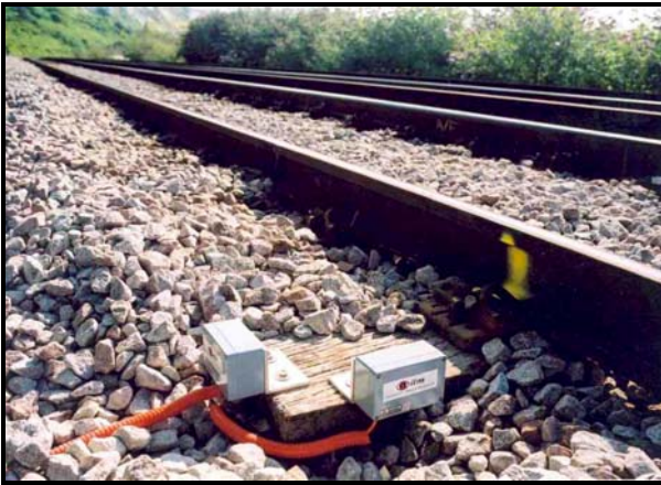
Figure 7. Tiltmeters measure real-time deflections.
