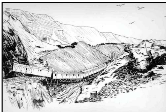
Figure 2. View east of the major slip in 1915.
