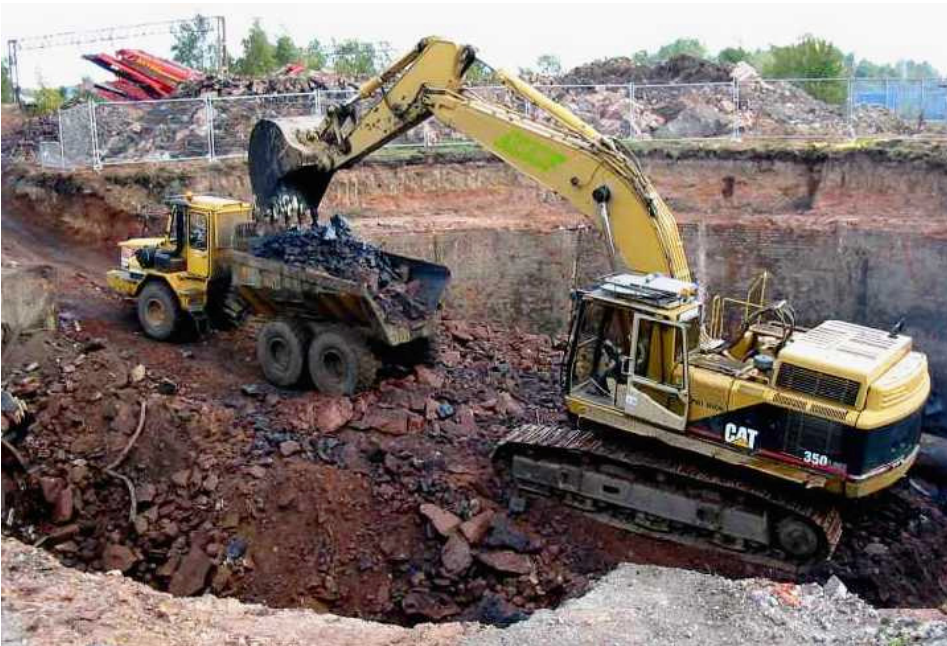
Figure 9. Excavation of a gasholder basin using a 50 tonne tracked excavator
