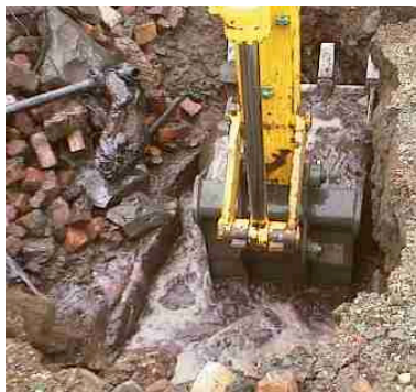
Figure 3. A combination of pink-tinted phenolic liquor, water and backfill material within a subsurface chamber
