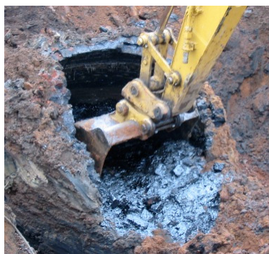
Figure 2. A chamber containing a coal tar backfill mixture placed originally during plant demoliton.
