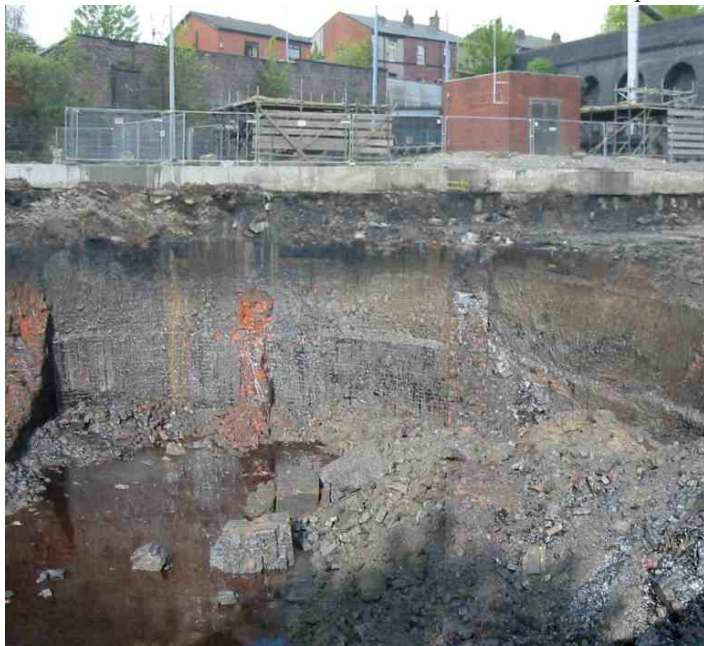
Figure 8. Tar well partially excavated
