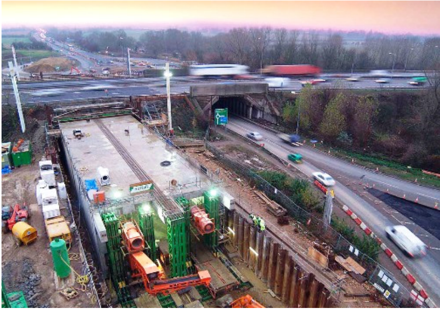
Figure 9. Partially installed underpass box
