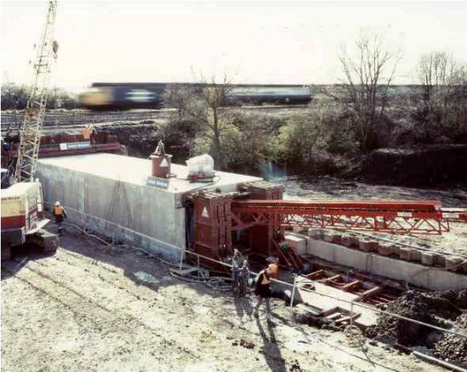
Figure 5. Subway box half way into embankment
