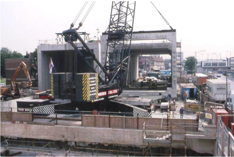
Figure 7. Tunnel segments at ground level in constricted site
