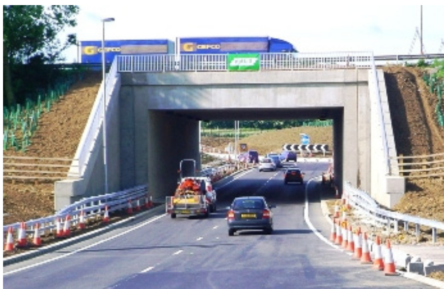
Figure 11. Underpass in use
