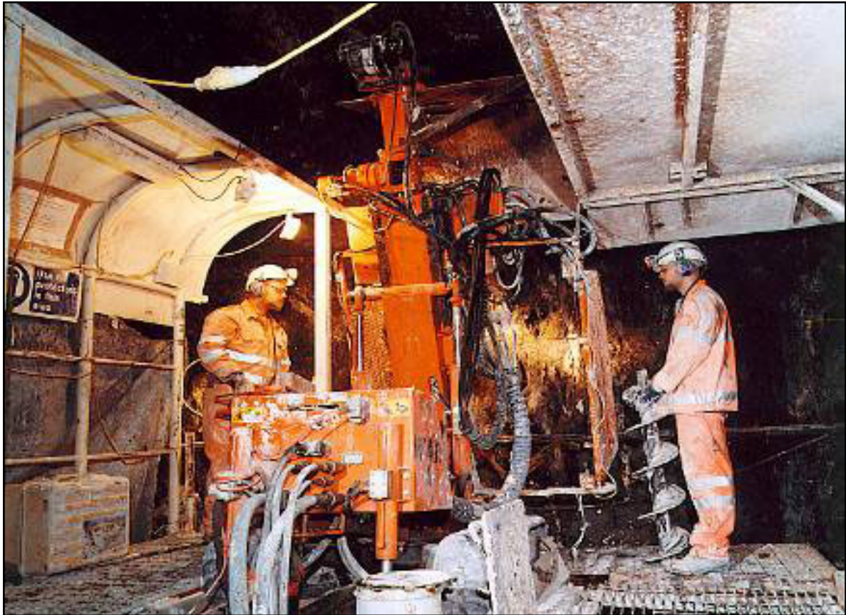
Figure 9. Auger rig used for piling operations
