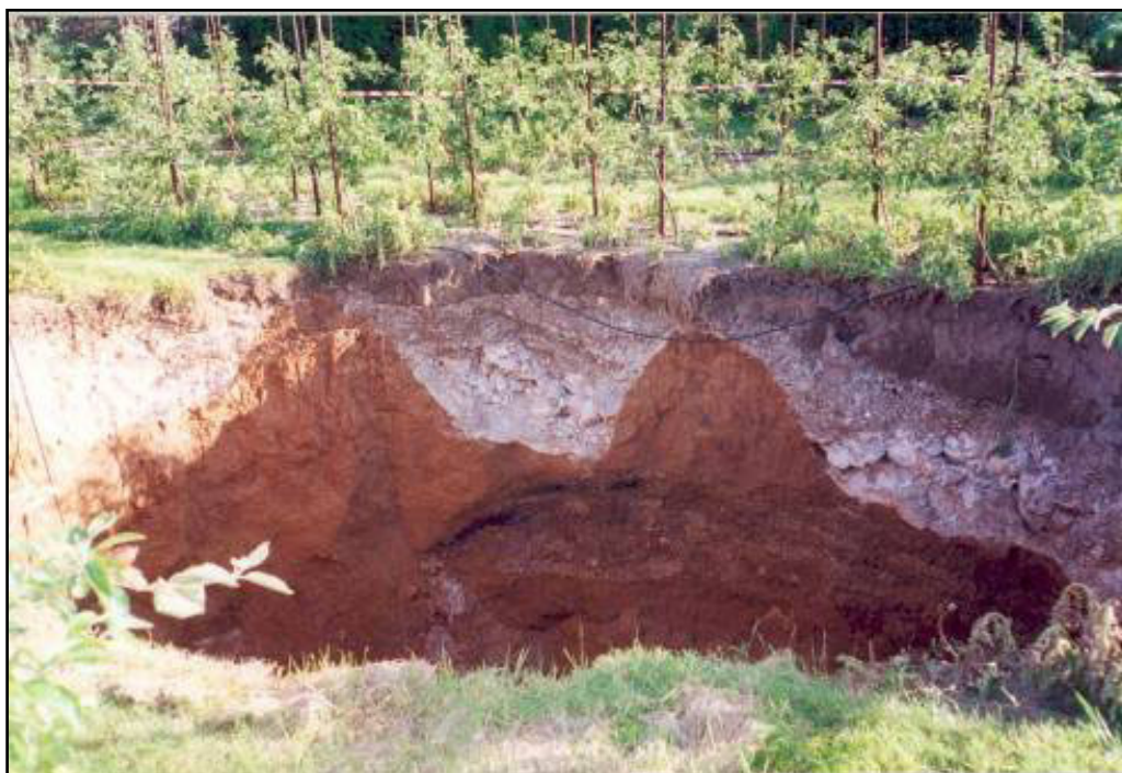
Figure 6. Surface void produced by collapse of shaft S4
