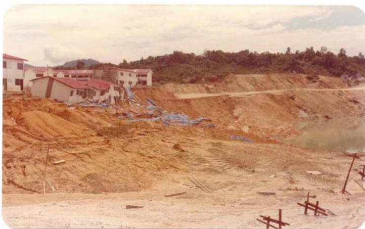
Figure 3. Slope failure due to dewatering of ex-mining pond, Cheras, Kuala Lumpur.
